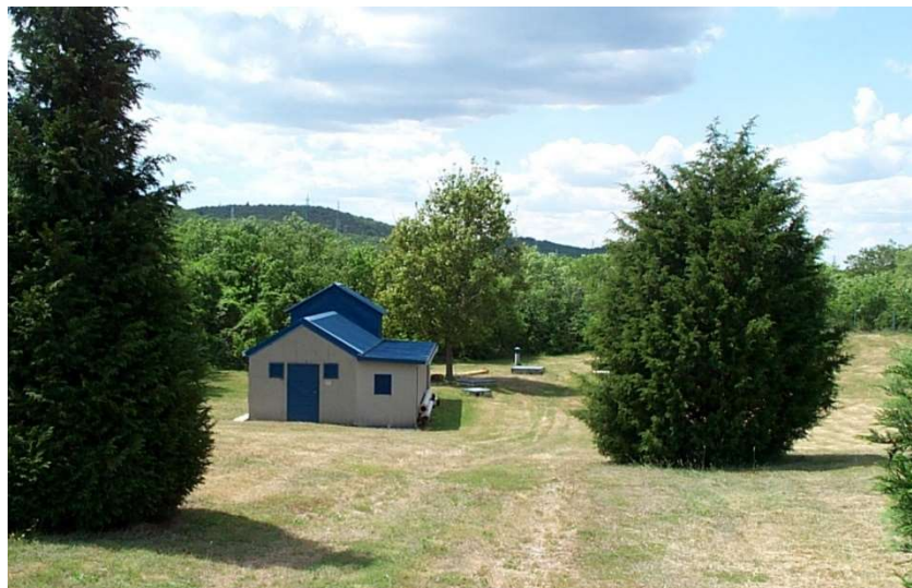
Figure 37: Drinking water pumping station Klariči
